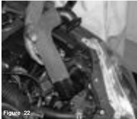
Figure 22 The entire air resonator air duct is now removed from the fender wall as shown above.
