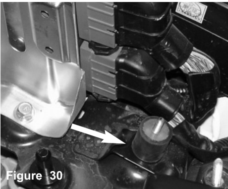
Figure 30 The vibra-mount is installed.
