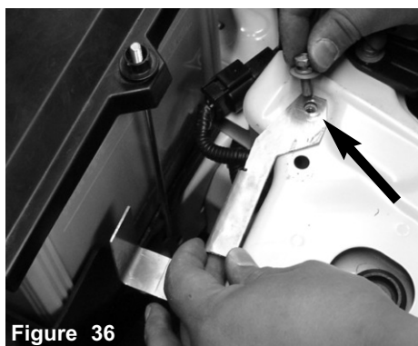
Figure 36 The stock 10mm bolt is used to secure the new fuse box bracket.
