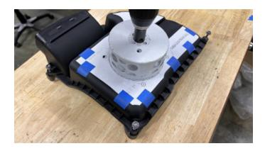
**36.** Once all the holes are drilled, remove the template. This is how the lid should look now.
